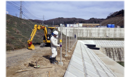
Disaster prevention regulating pond reinforcement work
