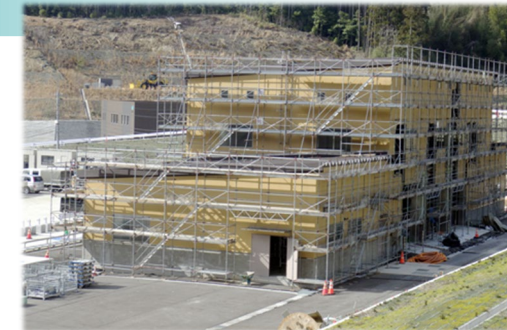
Leachate treatment facility outer wall repair work
