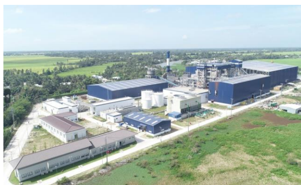
Hau Giang Biomass Power Plant
