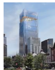
TOKYO TORCH (B棟)
