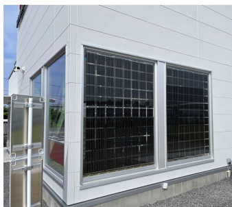
Installation of solar glass
